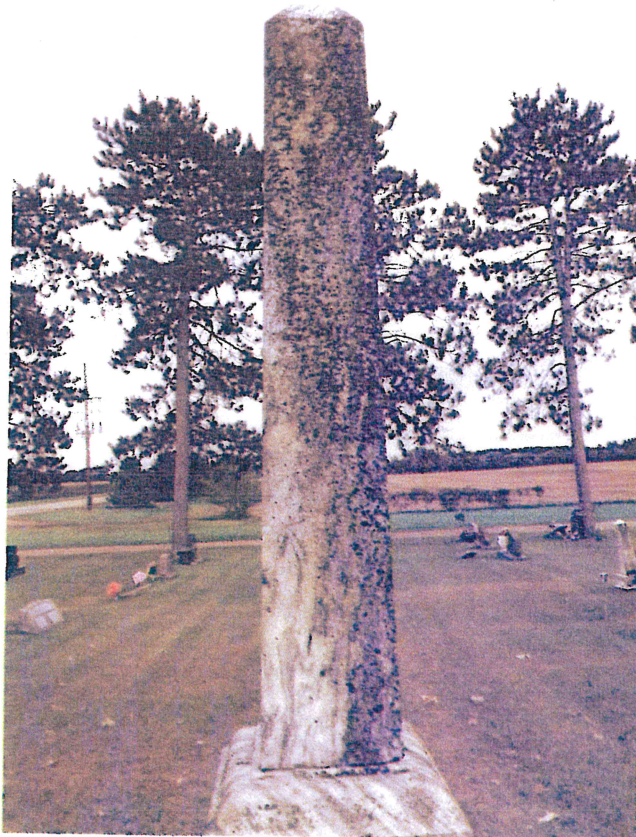
Left-Before cleaning and restoration.
